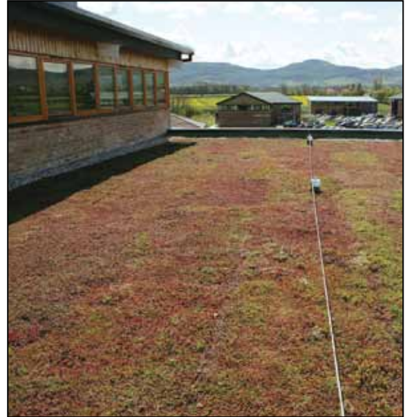
Green Roof at Momentum Business Centre
